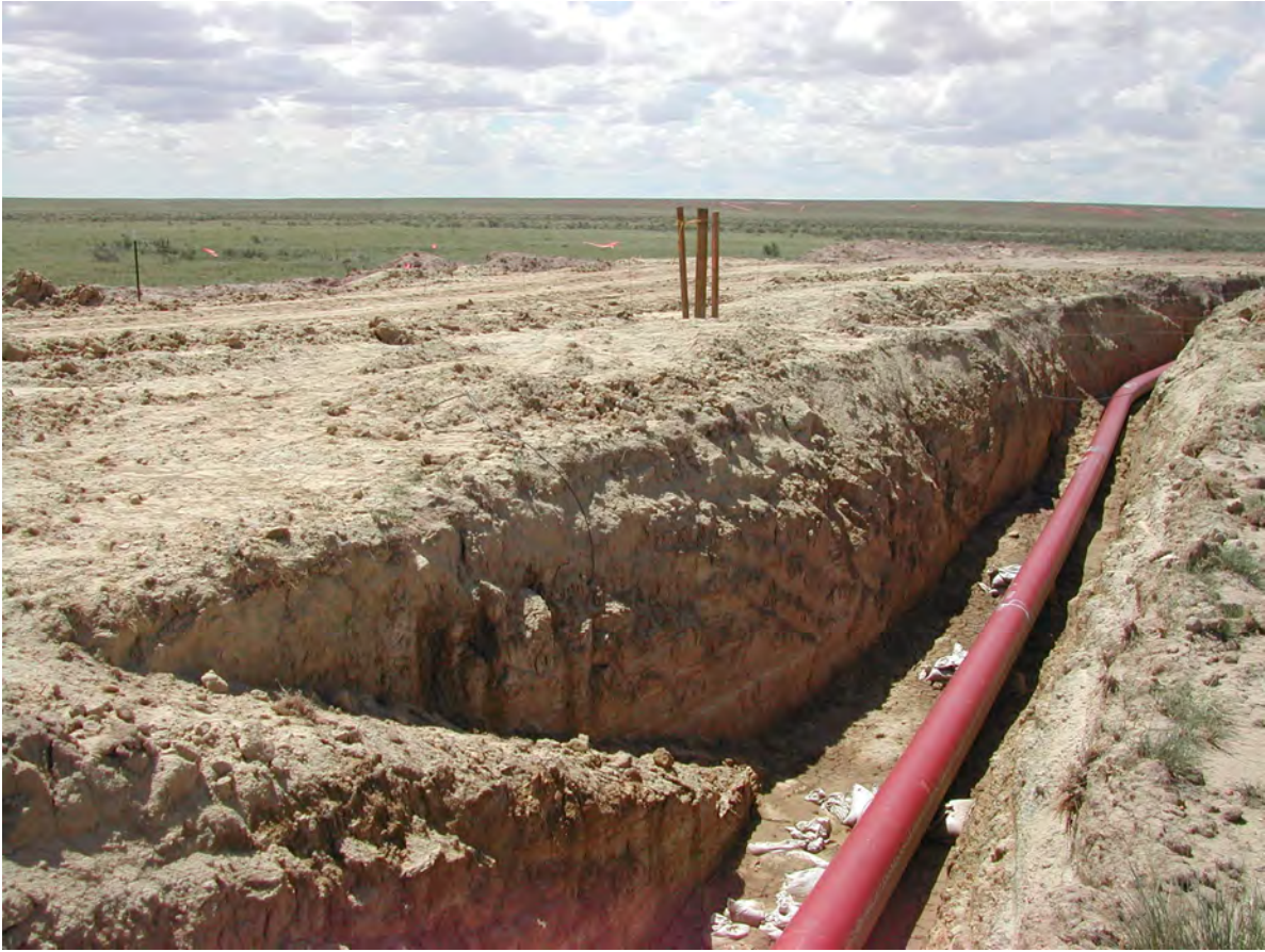
Escape ramps allow trapped wildlife to leave the trench. Photo M. Watson.
